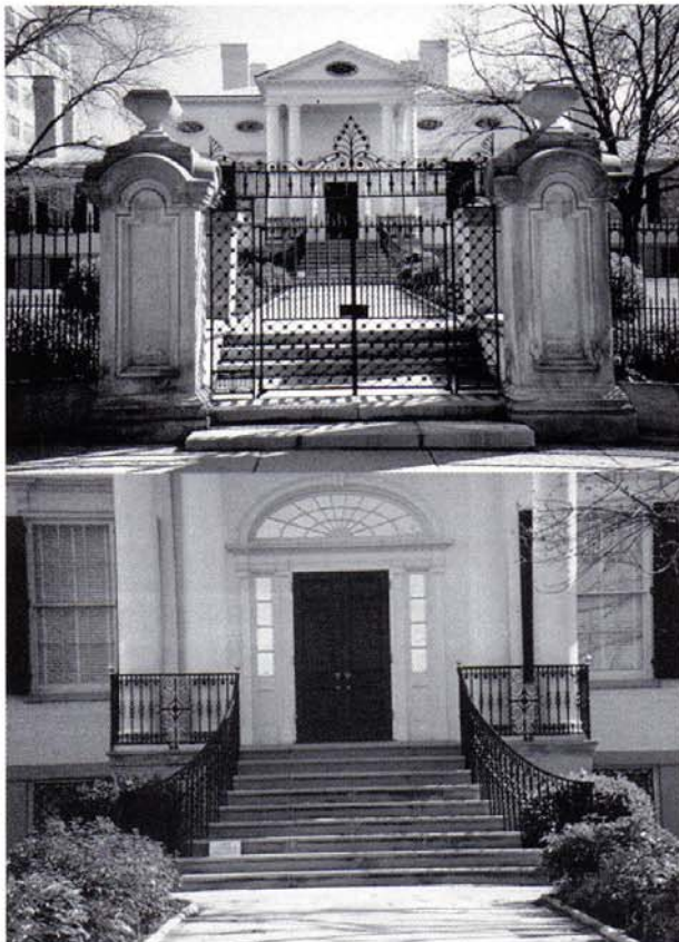
• Finished restoration of ornamental iron fence, gates, and railing at the Taft Museum, Cincinnati, OH. The original ironwork was also fabricated by Stewart Iron during the late 1800's.
